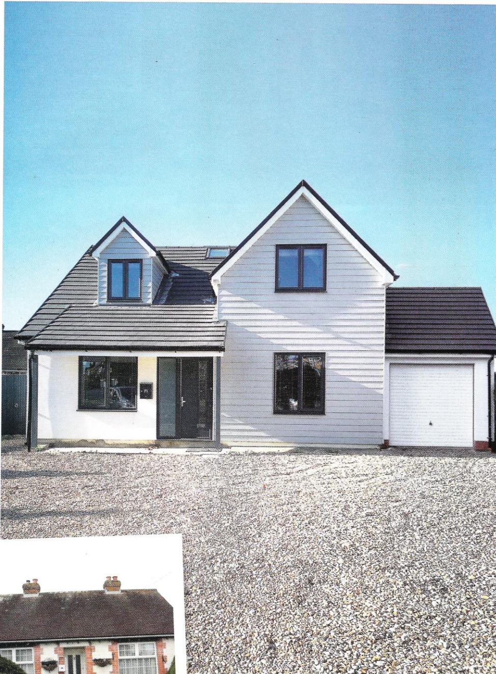
ABOVE Space & Style Home Design extended a small pre-war bungalow in Fareham, Hampshire, up and outwards for £230,000 and it now has three bedrooms. Big gables, an open porch, a widened entrance, cladding and self-coloured render give the building a New England look. Window and door openings were adjusted to suit the new design.
